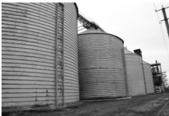
Figure 6 – Spiral-fold silos (elevator in village Emylivka, Kirovohrad region, 1971)
