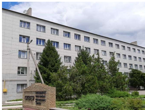
Figure 1 – An example of successful facade thermal modernization
