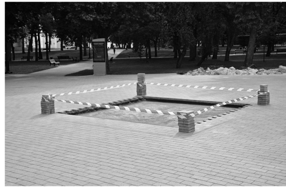
Figure 7 – Concrete preparation under the pedestal for the model in Chernihiv [12]
